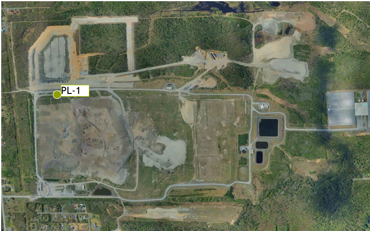
Station de pompage
